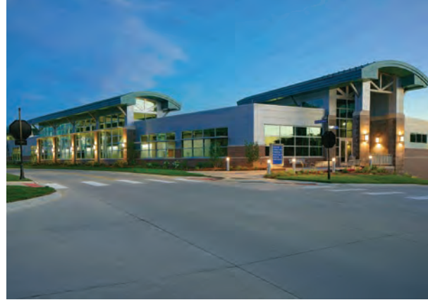
Kinney Hall at Iowa Western Community College
