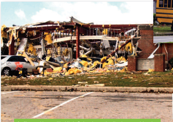
Indiana. Henryville High School was badly damaged by the storms. Photo by Dan Goldblatt/Indiana Public Media News
