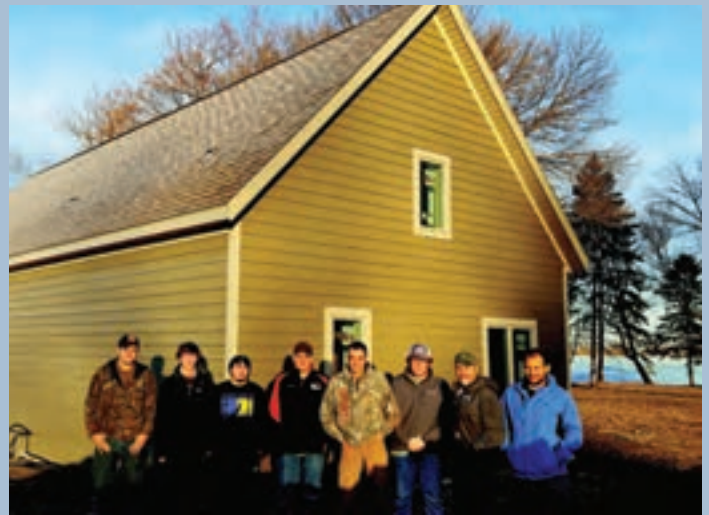
Iowa Lakes' Five Island Lake Cabin project
