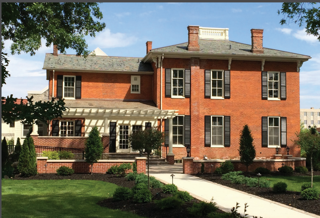
Heidelberg University Honors Program. Bryenton Center for Honors renovation.
