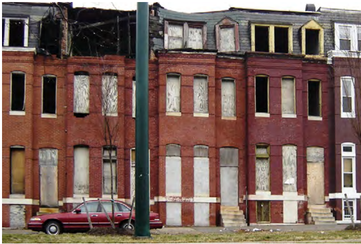
Renovation of homes on Broadway, before and after.
