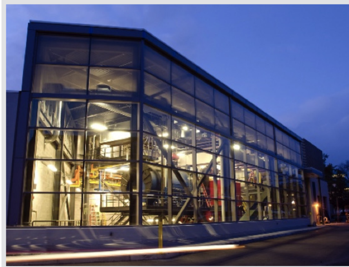
Middlebury College's $12 million biomass gasification plant moves the college closer to carbon neutrality.
