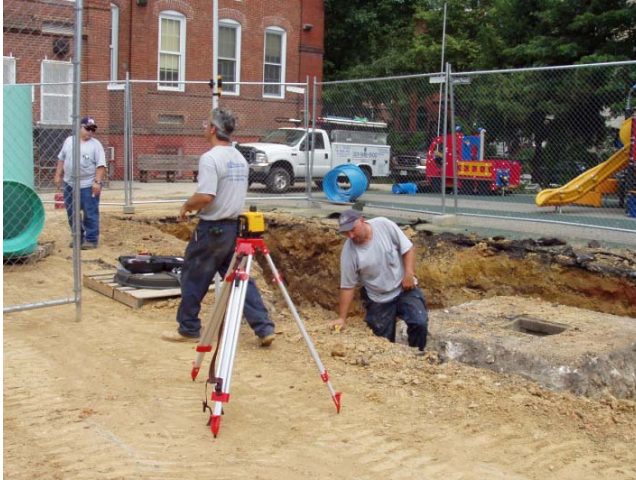
Measuring for Accuracy Ross Elementary School
