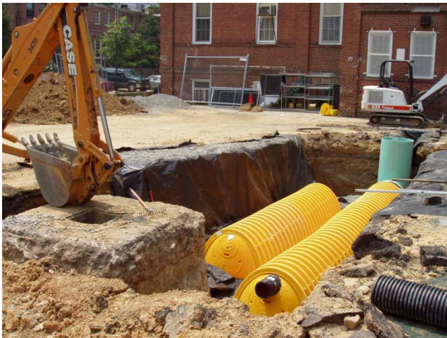
Underground Storm Water Control Ross Elementary School
