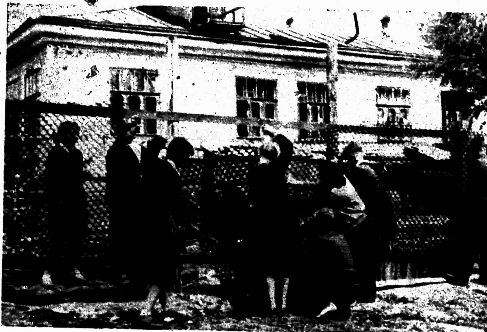
Figure 2-4.—"Socially useful work" at rural school. Building a rabbit pen.
