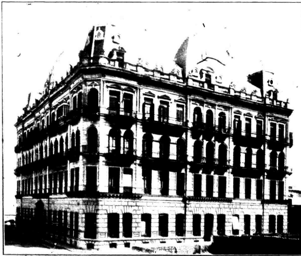
2. OLD UNIVERSITY BUILDING, NOW USED FOR THE SCHOOL OF ENGINEERING, MONTEVIDEO, URUGUAY.
