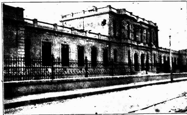
II. REAR VIEW OF THE SAME BUILDING.
