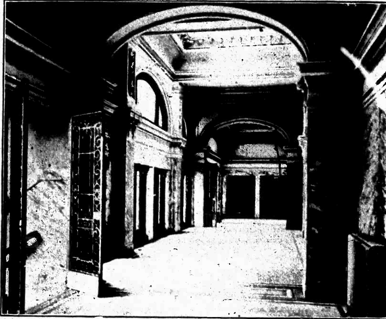
A. FOYER, DE WITT CLINTON HIGH SCHOOL, NEW YORK CITY. C. B. J. SNYDER, ARCHITECT.
