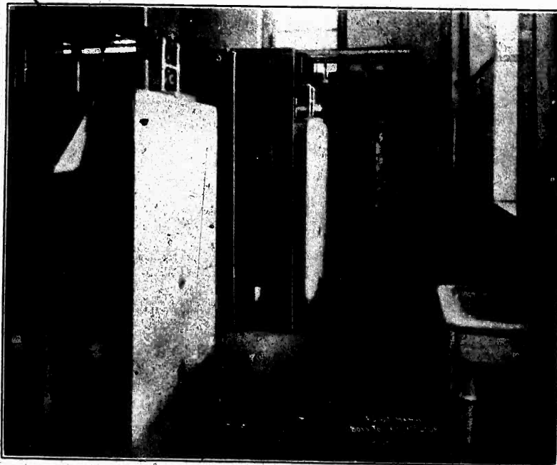
BOYS' TOILET ON THIRD FLOOR, PUBLIC SCHOOL NO. 62, NEW YORK CITY. INDIVIDUAL WASHOUT TANKS ARE PROVIDED.
