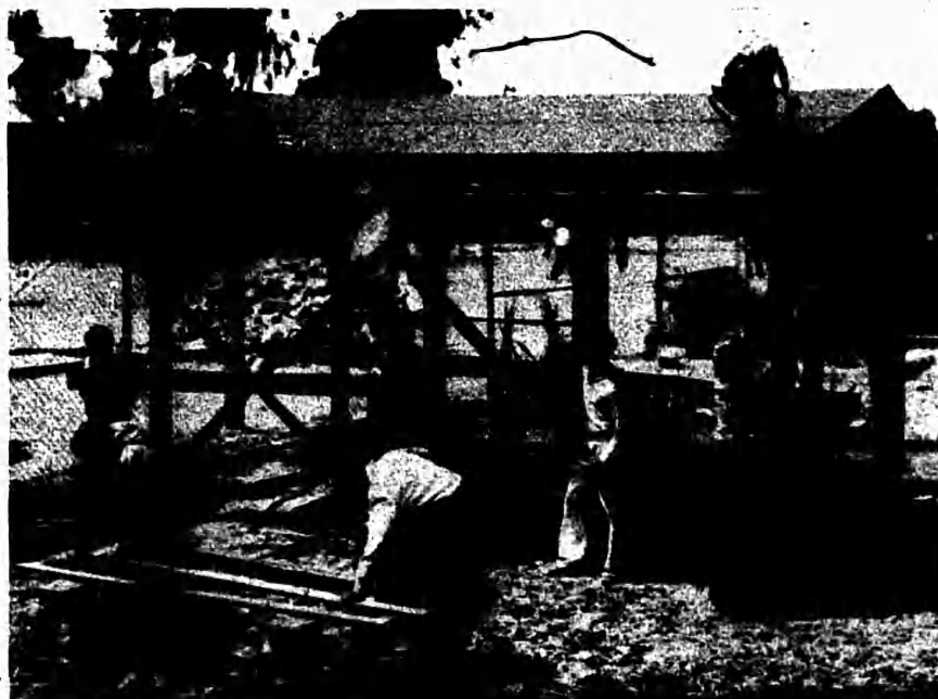
Erecting a farm building on the school grounds.
