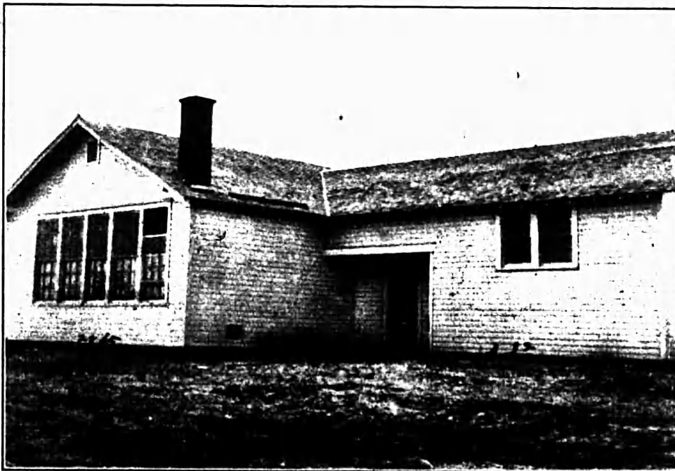
B. ALL OUTSIDE DOORS SHOULD BE PROTECTED BY AN OPEN VESTIBULE FROM TROUBLES DUE TO WIND AND RAIN
