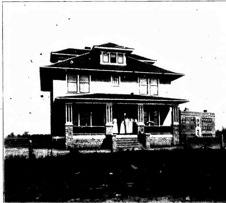
II. TEACHERS' COTTAGE, ROLLO CONSOLIDATED SCHOOL.
