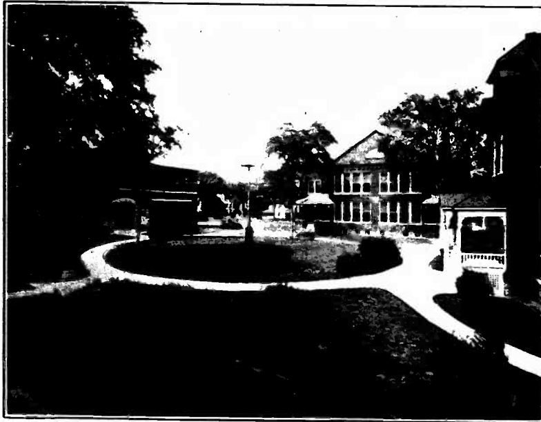
A. SCHOOL DECORATION. SCHOOL GROUNDS, HUDSON FALLS, N. Y. (Courtesy of University of State of New York.)
