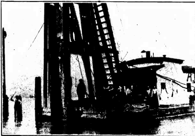
B. A PILE DRIVER NEAR METLAKATLA.
