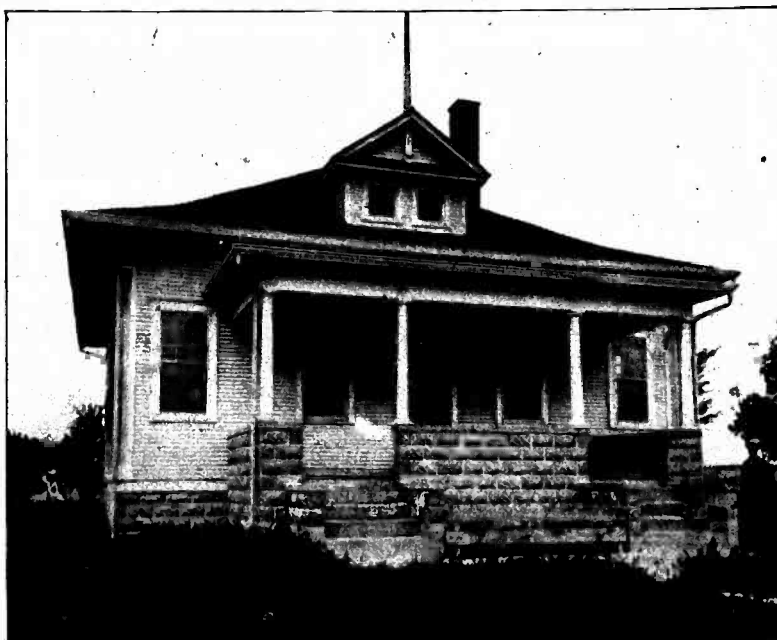
B. A NEW RURAL BUILDING STANDARD IN ALL RESPECTS. IN COLFAX COUNTY.
