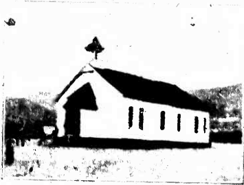
C. A FRAME STRUCTURE AT CHLO- RIDE, MOHAVE COUNTY.
