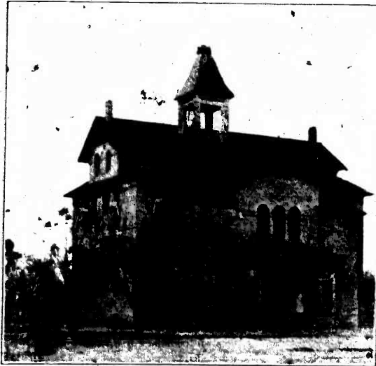
A. THE OLD SCHOOL BUILDING NEAR WHICH NEW UNIT BUILDINGS HAVE BEEN CONSTRUCTED.
