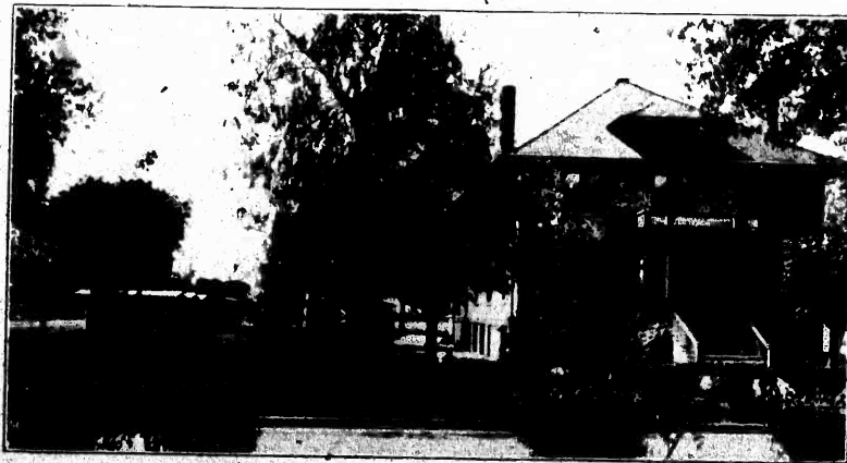
C. BOYS' DORMITORY AND OVERFLOW COTTAGES.
