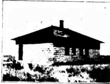
B. A CONCRETE BLOCK BUILDING IN COCHISE COUNTY.
