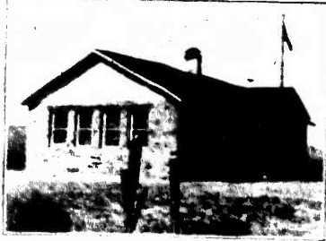
A. A TWO-ROOM BUILDING IN YAVAPAI COUNTY.
