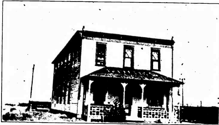
A. OLD ROOMING HOUSE TRANSFORMED INTO A DORMITORY, STANFORD, MONT.
