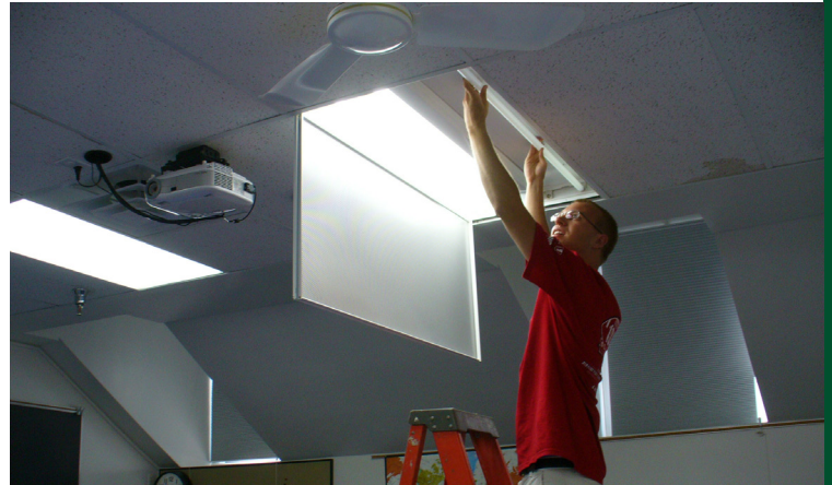
The College of Saint Benedict and Saint John’s University in Minnesota share a GRF. In the summer of 2012, the College of Saint Benedict underwent a campus-wide lighting upgrade to update college buildings from 35W four foot lamps to 25 Watt lamps. The project cost $50,000, $15,000 of which went to 3 student employees who carried out the upgrade. The project is estimated to have an annual savings of 715,000kWh, the equivalent of approximately 425 tons of carbon per year. The college estimates a project payback of about a year.
