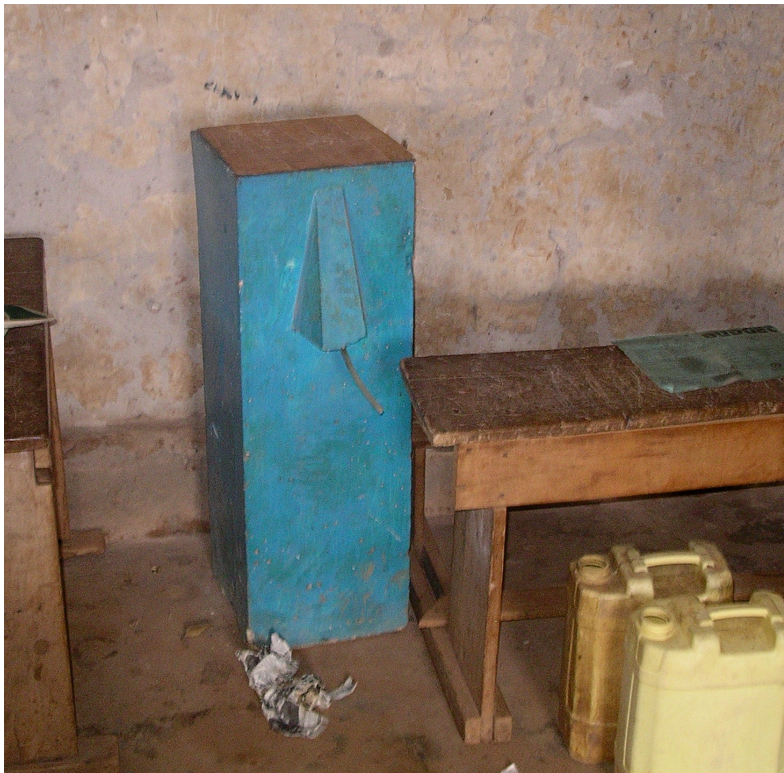
Figure 8: BSF at St. Paul's School shows effluent tube.
