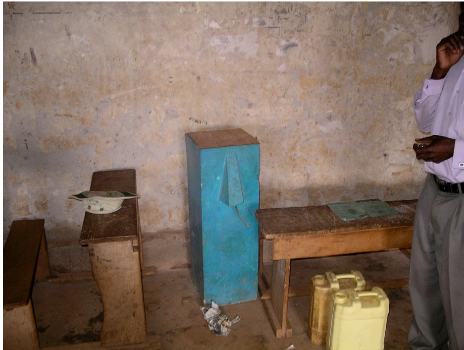
Figure 1 Biosand filter at St. Paul school in Nkokonjeru, Uganda. Notice the yellow plastic jerry cans.
