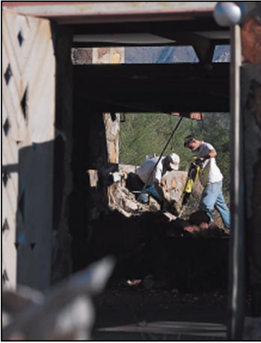
As part of the “hands-on” educational approach at the Wright School, students wield a jackhammer in the early stages of expanding a computer lab.
