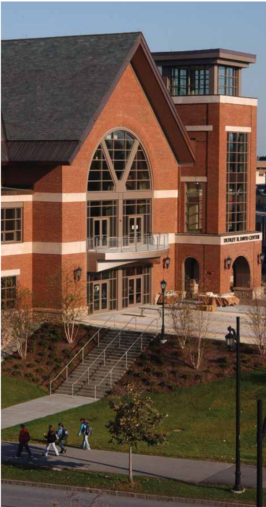
■ The LEED-Gold certified Davis Center at the University of Vermont opened in 2007.
