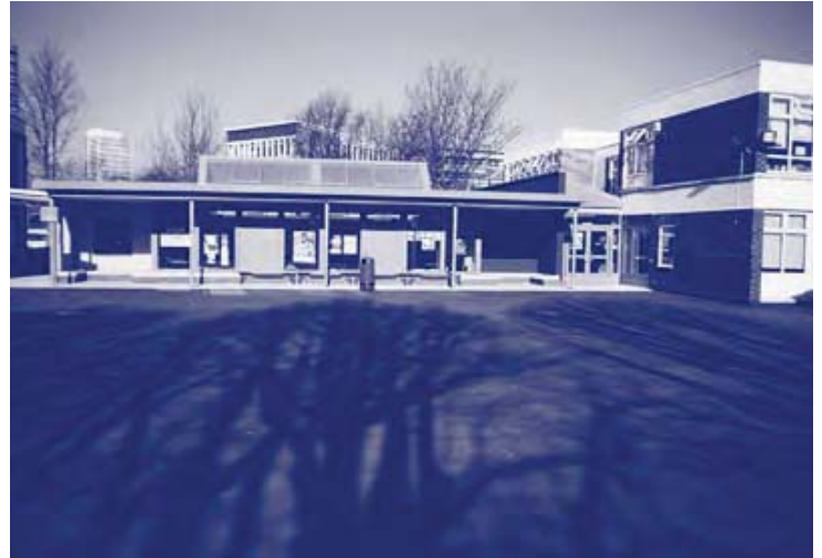
External view of the learning resource centre with alcove seating
