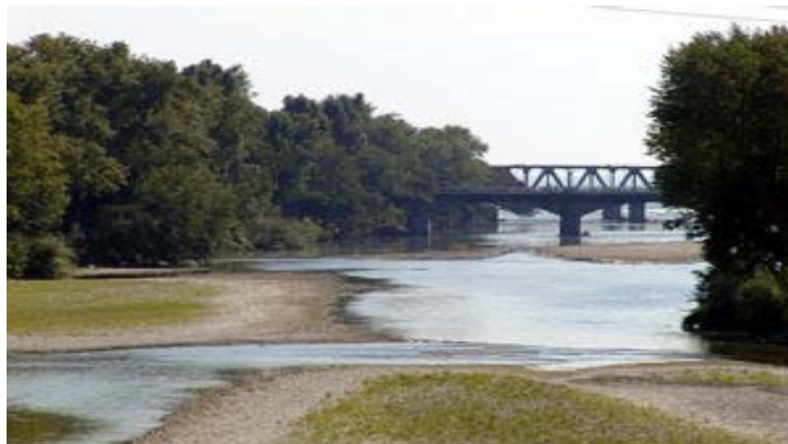
Figure 1. The river Entella: Railway bridge.
