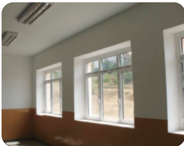
Rehabilitated classroom at Kiril i Metodij School in Bosilovo, Macedonia
