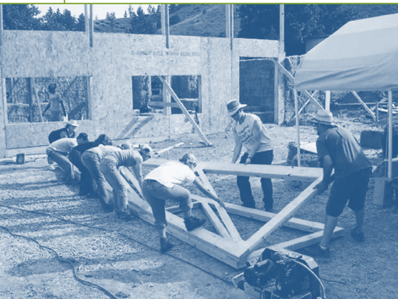
Early Childhood Learning Center under construction.
