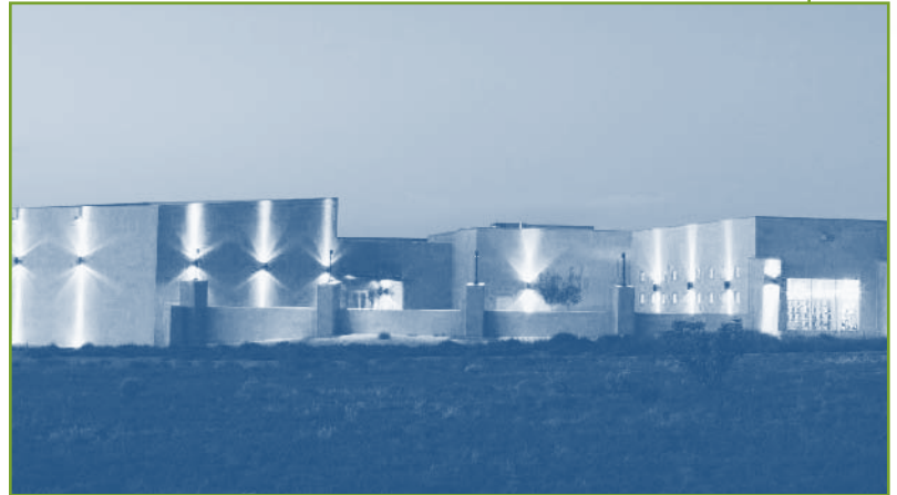
Library and Technology Center at IAIA.
