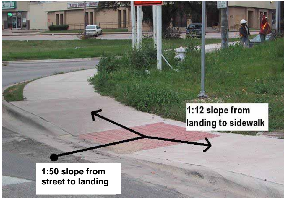
Figure 8-16. Photo. Parallel curb ramp.
