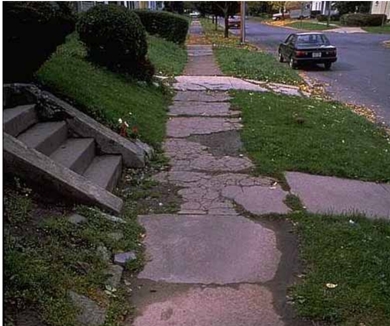
Figure 22-1. Photo. Courts have become less sympathetic to agencies that do not consider the needs of pedestrians and bicyclists.
