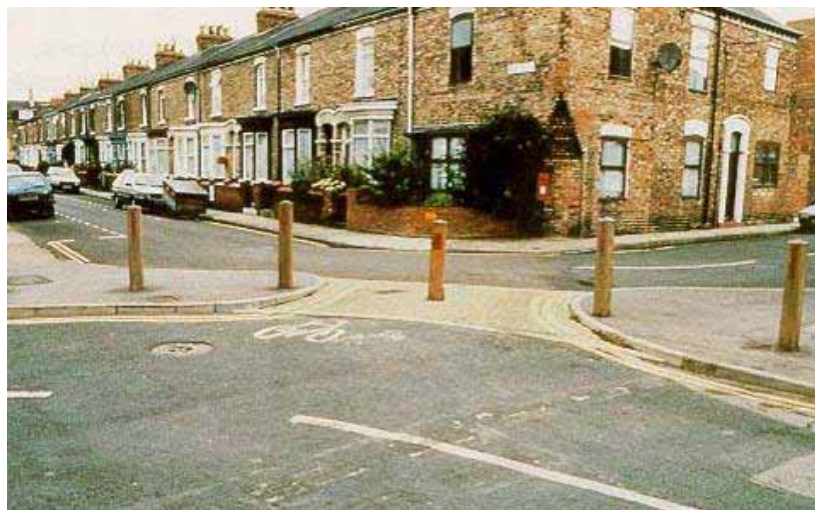
Figure 20-14. Photo. Diagonal road closures/diverters limit vehicular access but allow emergency vehicles to enter through removable bollards.
