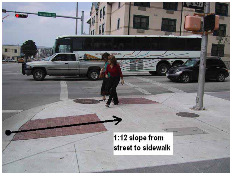
Figure 8-15. Photo. Perpendicular curb ramp.
