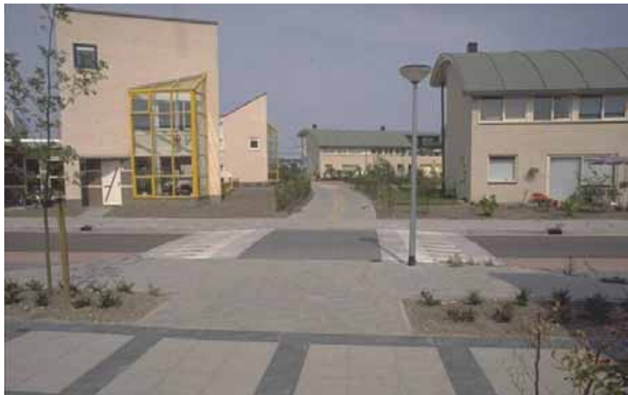
Figure 20-7. Photo. Raised crosswalks can slow traffic and give pedestrians a level surface at the crossing.
