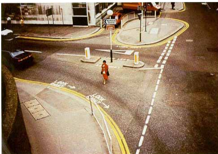
Figure 10-7. Photo. “Look Right” or “Look Left” is painted on the street next to the curb in the United Kingdom.
