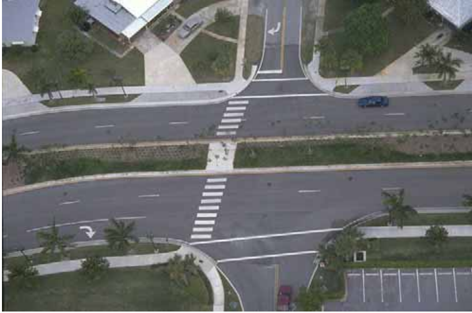
Figure 11-16. Photo. Refuge islands provide pedestrians with a resting place when crossing roads or intersections.
