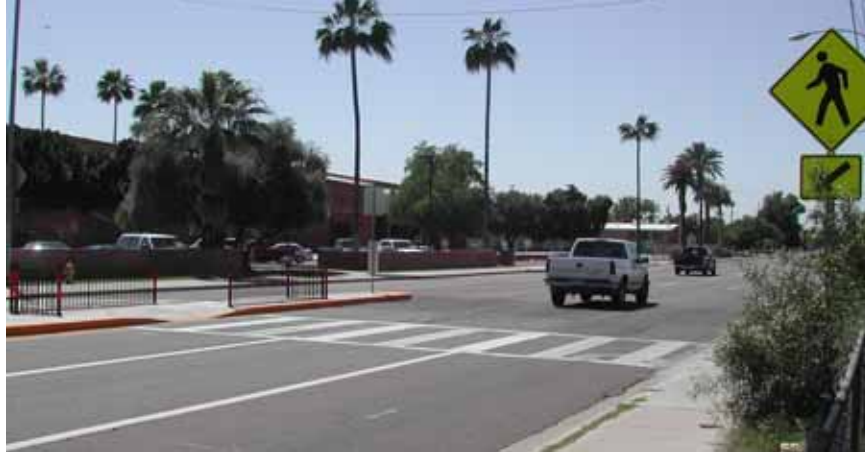
Figure 20-9. Photo. This median refuge island provides railing and a staggered crossing area to direct pedestrian views toward oncoming traffic.
