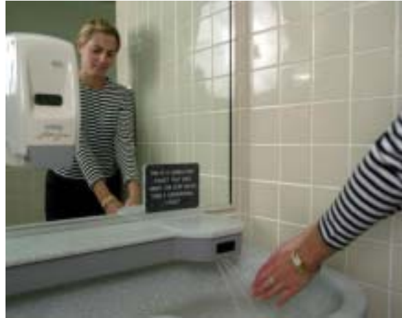
Low-flow devices will reduce water consumption by 15% to 20%, resulting in lower environmental costs and reduced load on wastewater treatment plants. NREL/PIX00653
