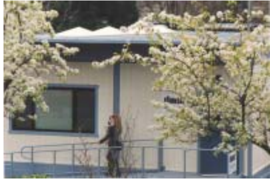
Pyramid skylights on experimental portable classroom design integrate skylights into a high efficiency modular design. NREL/PIX 11400
