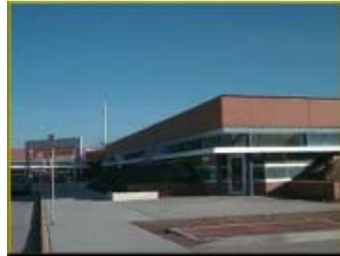
Exterior lightshelves reflect sunlight onto classroom ceilings. NREL/PIX 11435
