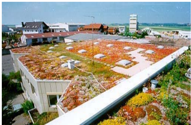
A vegetated roof reduces the amount of rainwater runoff while simultaneously minimizing heat build-up and providing insulation.
