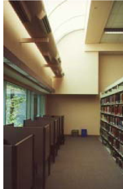
View windows are separated from the daylight feature overhead and use lower transmission glass to reduce glare.
