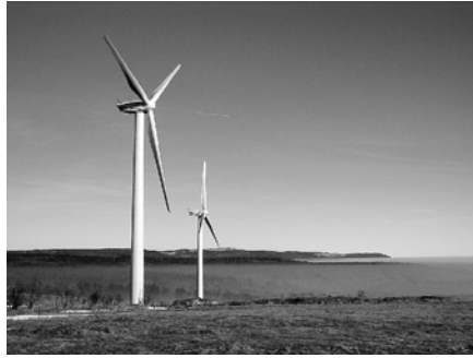
Figure 5 Wind power station in Nova Ves
