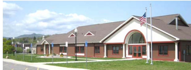
The new Ticonderoga campus of North Country Community College
