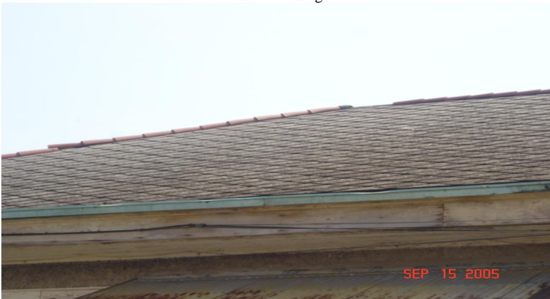
Roof ridge tile damage
