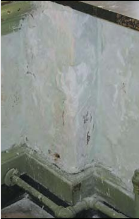
Age and neglect have left the walls in some schools—like this New York classroom—literally crumbling.
