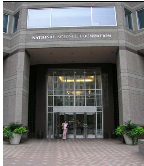
National Science Foundation entrance
