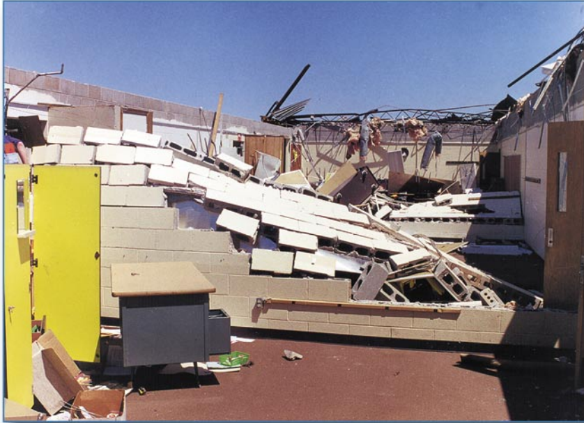
Figure 6-34 The interior walls of this classroom wing were constructed of unreinforced CMU.
