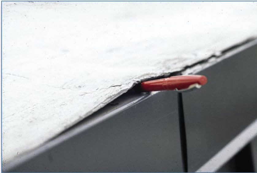
Figure 6-37 The metal edge flashing on this modified bitumen membrane roof was installed underneath the membrane, rather than on top of it and then stripped in. In this location, the edge flashing is unable to clamp the membrane down. At one area, the membrane was not sealed to the flashing (an ink pen was inserted into the opening prior to photographing). Wind can catch the opening and lift and peel the membrane.
