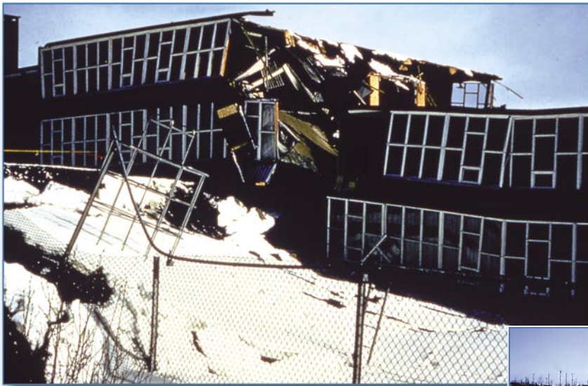
Figure 4-1 School, Anchorage, AK, 1964, severely damaged by earthquake-induced landslide
