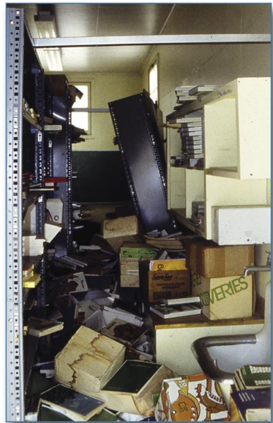
Figure 4-10 Fallen filing cabinets and shelves, Northridge, CA, 1994
