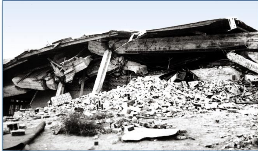
Figure 4-8 Collapse of portion of nonductile concrete frame school structure, Helena, MT, 1935
