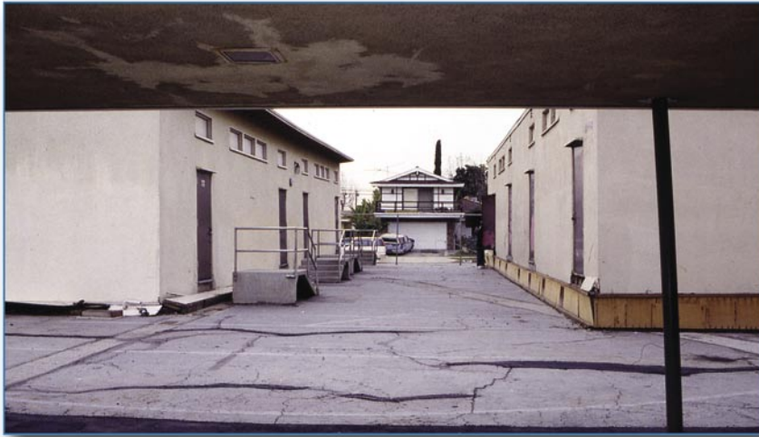
Figure 4-9 Modular classrooms pushed off their foundations; note stairs at left, Northridge, CA, 1994.
