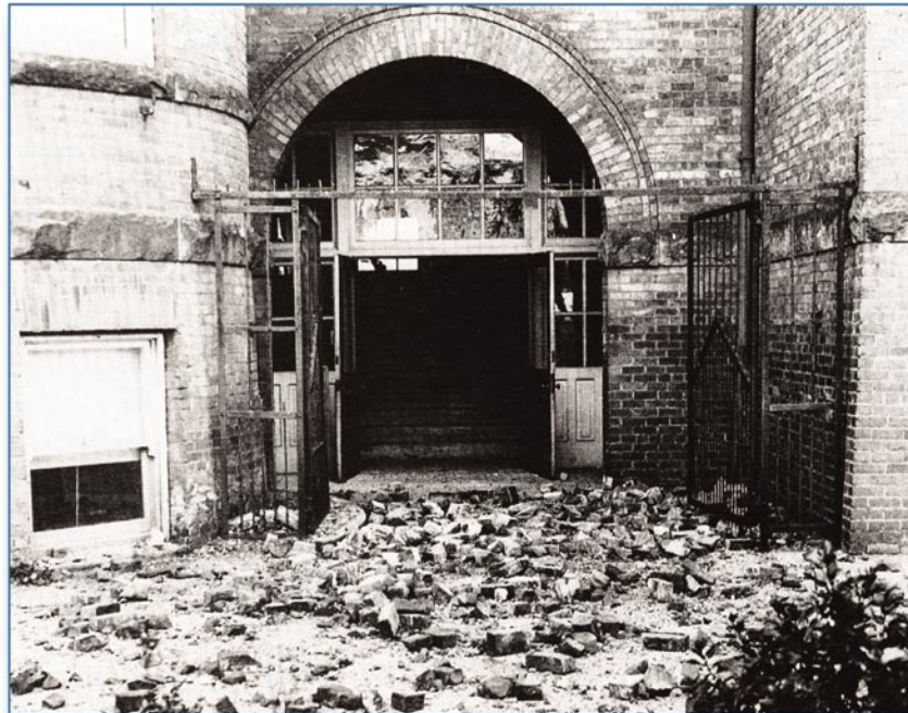
Figure 4-22 Another dangerous entry collapse, Seattle, WA, 1949
