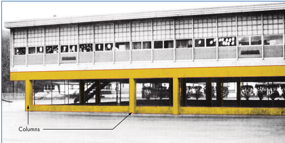
Figure 5-6 Elementary school in Jefferson County, OH, elevated on columns
