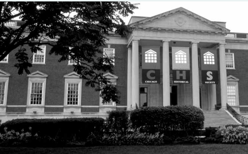
East facade of the Chicago Historical Society , the original 1931 entrance, that faces out on Lincoln Park.
