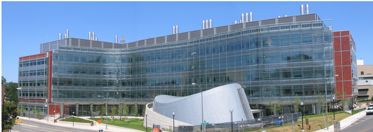
University of Michigan's New Biomedical Research Building iii
