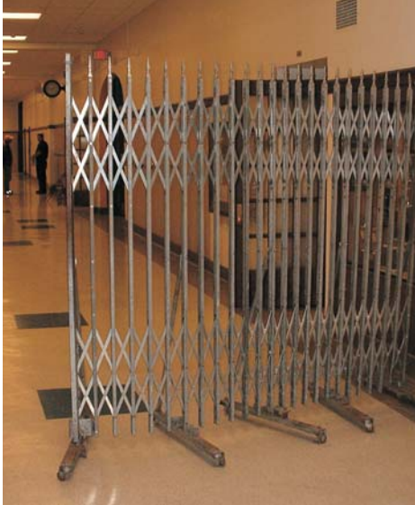
Barriers such as interior gates can help keep unauthorized persons out of areas vulnerable to theft or vandalism after hours.
