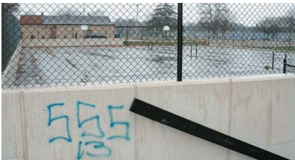
Graffiti tagging and other forms of defacement often mark school buildings and grounds.
