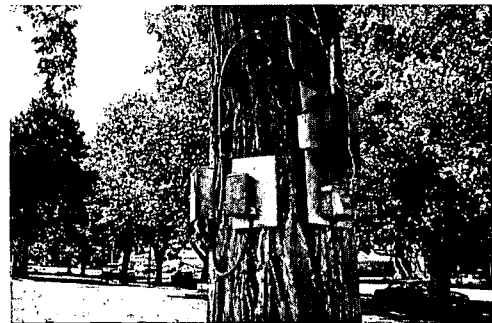
Exterior lighting and power
