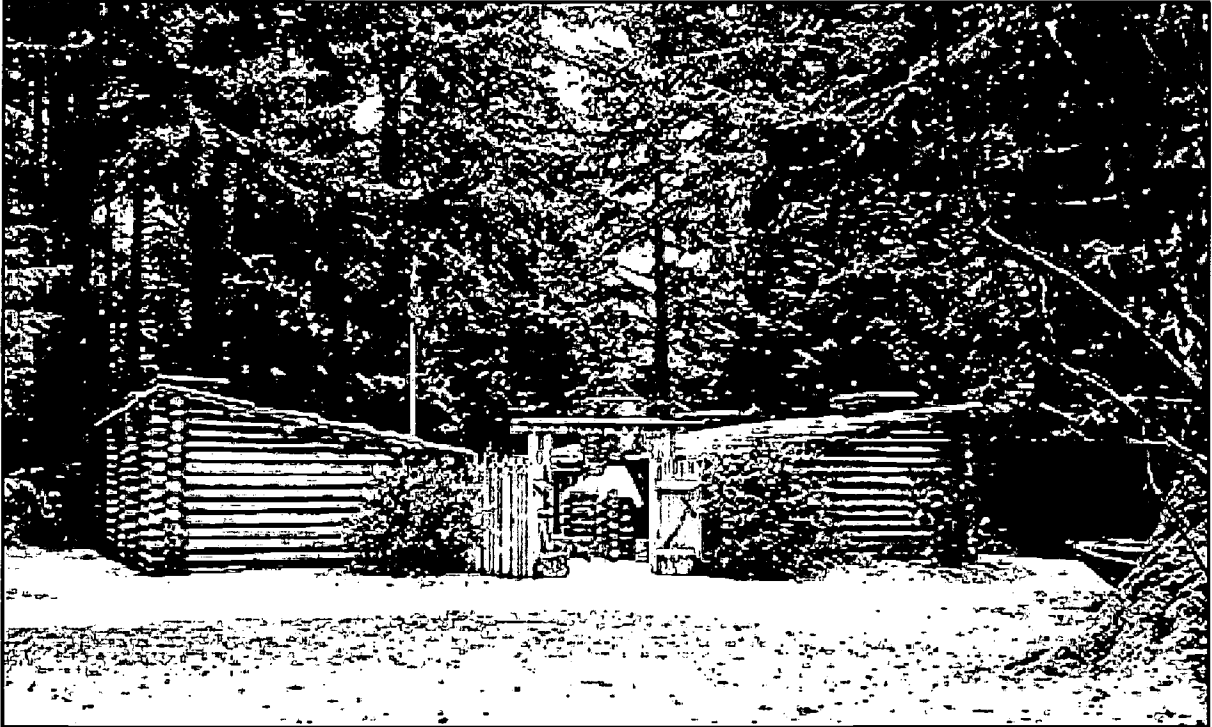
(National Park Service, Fort Clatsop National Memorial)
