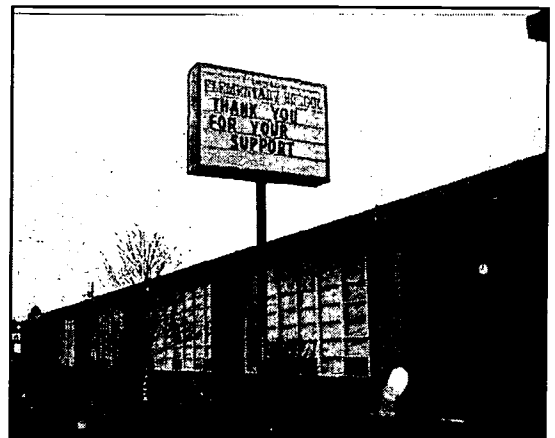
Stayton Elementary School and Stayton Middle School students, teachers and staff benefited from lighting and heating/cooling system improvements.
