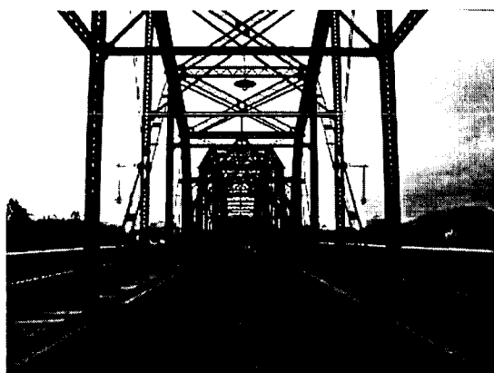
Walnut Street Bridge
