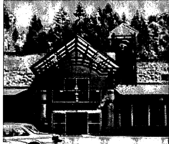
CMU Construction at the Central Market, Poulsbo, Washington. Photo courtesy of O'Brien and Co, Inc.
