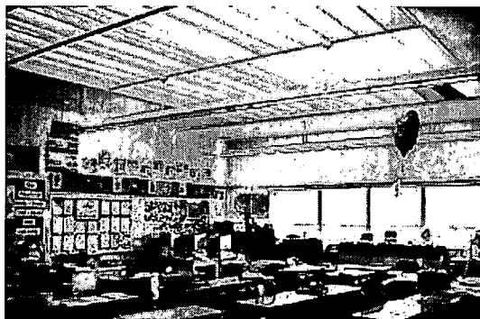
Gentle, diffuse daylight permeates a classroom with both sidelight and toplight. Note that all surfaces are painted white to distribute light more efficiently and reduce contrast glare. Photo courtesy Barbara Erwine.
