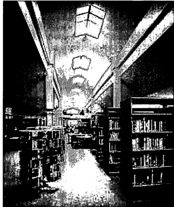
Linear skylight in this library spreads daylight to adjacent spaces and organizes the circulation
