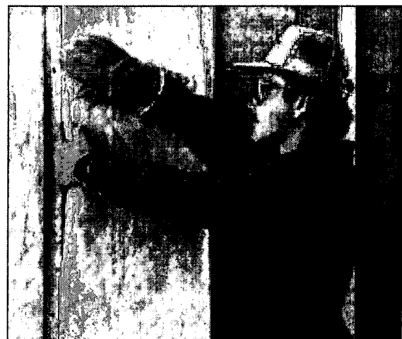
Masonry walls can be insulated on the interior, but the benefits of thermal mass are mostly lost. Photo Courtesy: CertainTeed.
