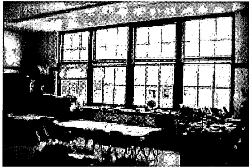
Large windows can create overly cold or warm surfaces, reducing thermal comfort. High performance glazing improves thermal comfort. Double glazing improves acoustic performance. Operable windows, which allow natural ventilation, improve student performance. (Photo courtesy Barbara Erwine)
