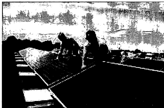
Photovoltaics are most cost effective in remote locations that are a distance from an electrical grid, but they have zero environmental costs. NREL/PIX07631.
