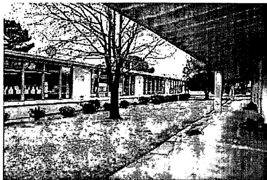
North versus south windows. South windows are shaded from direct sun, but receive daylight reflected off of concrete walk and white painted overhangs. North windows are large and unshaded. Photo courtesy Lisa Heschong.
