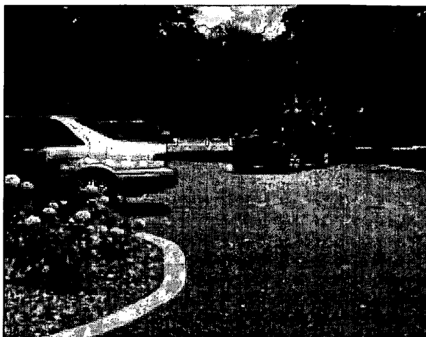
Student and Staff Parking at Dominican University, River Forest, Illinois. Made with Gravelpave porous paving, manufactured by Invisible Structures, Inc., Aurora, CO ( http://www.invisiblestructures.com ). A porous base course was constructed on top of existing site soils to leave tree roots undisturbed. 15" deep concrete curbs were installed with forms to curve around tree bases. The final top 1" of rings, grid and fabric were anchored in place to receive the gravel. Photo reprinted with permission from Invisible Structures, Inc.
