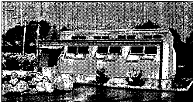
This relocatable structure is a prototype designed by Southern California Edison and contains high performance features such as daylighting, high indoor air quality, significant energy savings, and resource efficient materials.
