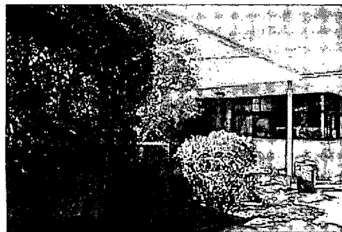
Overhangs and vegetation were designed to shade windows and prevent reflected glare. Curtains or blinds in windows provide additional control.
