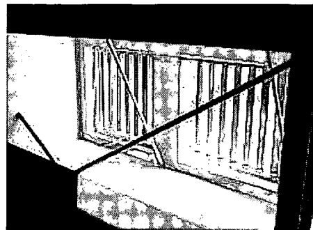
Operable louvers are not actively used. Photo courtesy Lisa Heschong.
