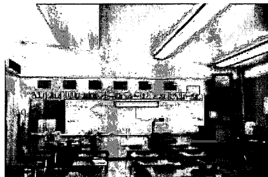
Lighting Controls, Oakridge High School: Automatic photosensor controls turn off first bank of lights next to skylight well. The light fixtures are arranged parallel to skylights to left and windows (out of picture) to right, while whiteboard is located perpendicular to windows and skylights. Photo courtesy Lisa Heschong
