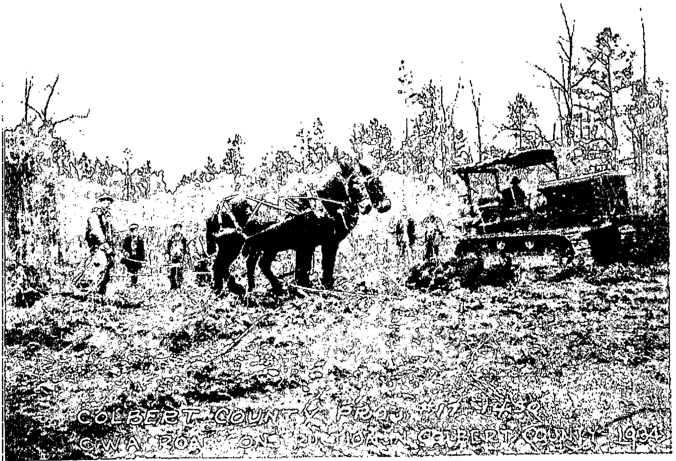
Road Construction in Colbert County
