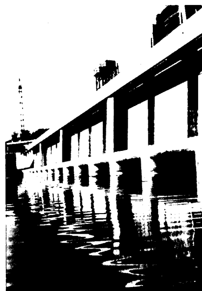
Tidal power generates electricity at the Rance Station on the northern coast of Brittany (France).
