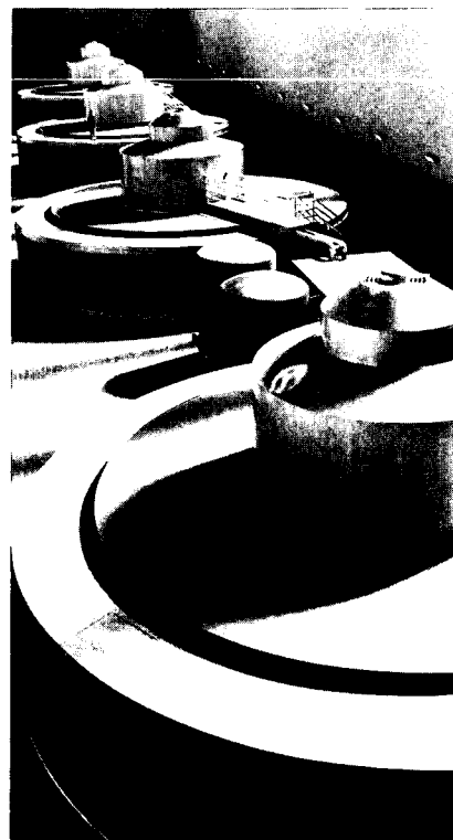
The energy produced by water flowing through dams is used to turn massive electric generators ( below right ) at hydroelectric plants such as this one at the Shasta Dam in California.
