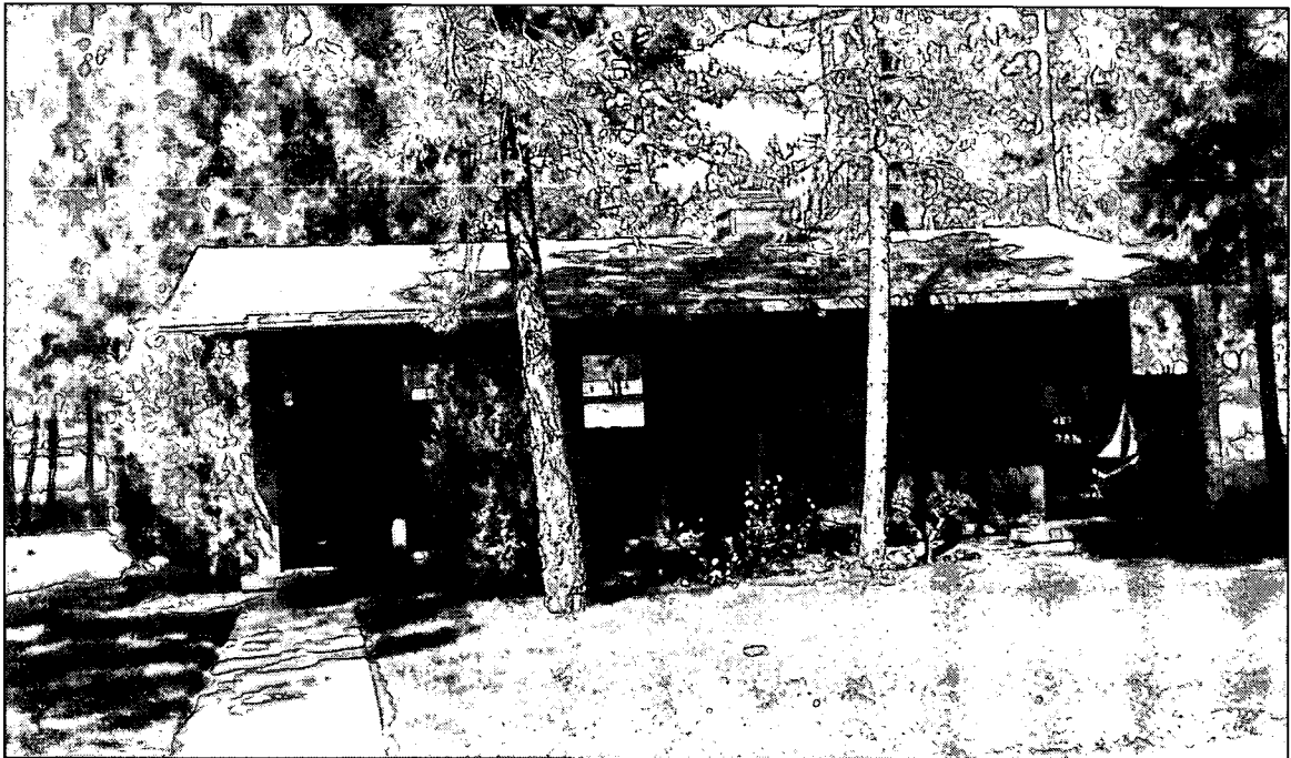
Kettle Falls Ranger Station, no date. This building was one of the first to be constructed at LARO, and it is still in use as a contact station. Photo courtesy of National Park Service, Harpers Ferry Center (HFC 64-155).
