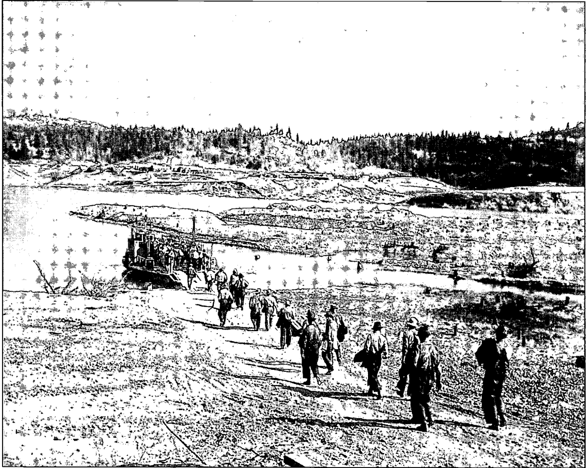
WPA workers boarding Gerome Ferry to take them to Camp Gerome, on the far side of the river. Note the tree stumps on the land that will be inundated by the reservoir. Photo courtesy of MSCUA, University of Washington (Grand Coulee Dam 5).
