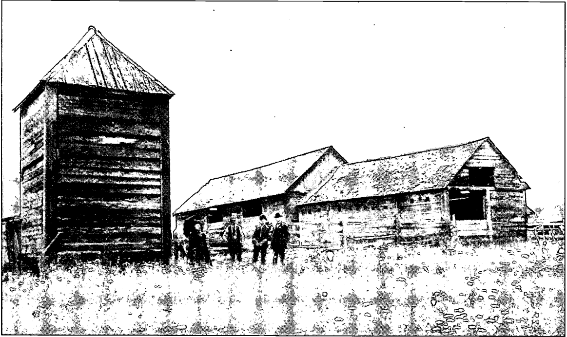
Fort Colville buildings, no date. Note the post-and-sill construction of the log structures. Photo courtesy of National Park Service, Lake Roosevelt National Recreation Area (LARO 2443).
