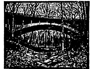
Ross Drive Bridge, Washington, DC.
