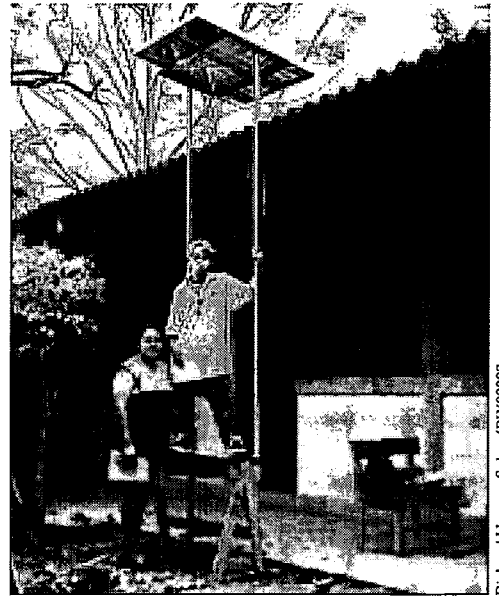
Figure 6.7. PV installation at Santa Cruz Minas.
