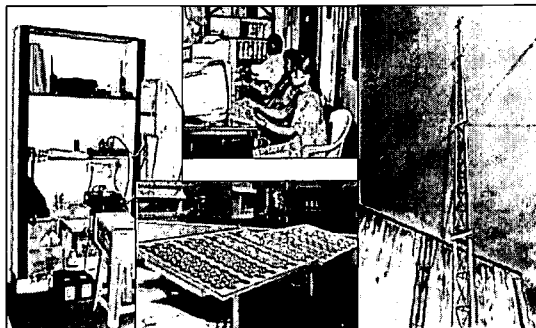
VHF two-way radio, Internet, Spread spectrum antenna and solar panels at Villianur
