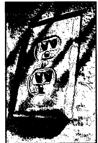
Grounding-type receptacle.
