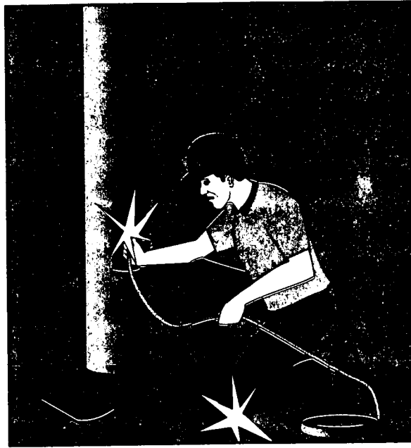
Worker was electrocuted while removing energized fish tape.
