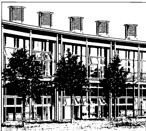
HAUTE VALLEE SCHOOL, JERSEY Stack ventilation through the 'chimneys' on the roof of the building keeps fresh air circulating around the school.
